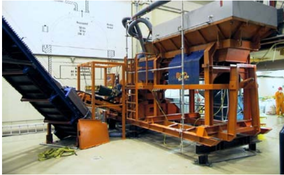
Concrete breaker at controlled area
