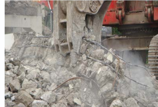
Crushing concrete structures
