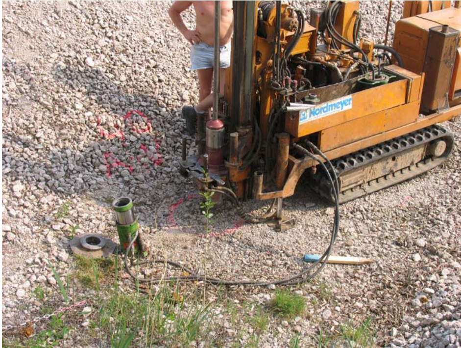
Drill core soundings on the site
