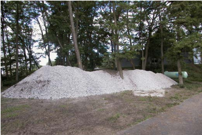
Intermediate storage of cleared concrete rubble
