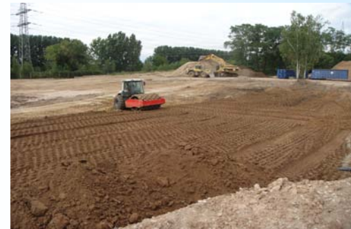
Preparation of soil surface
