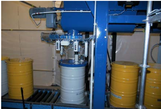
Filling of drums with concrete rubble
