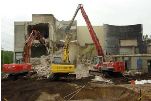
Demolishing waste treatment building
