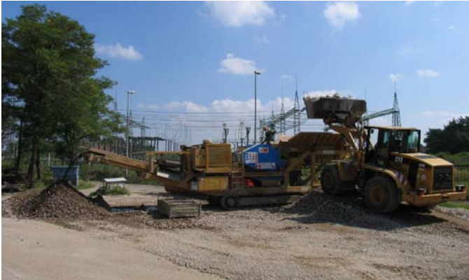
Concrete breaker unit
