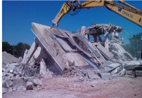
Demolishing turbine table
