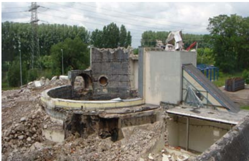
Lower part of reactor building
