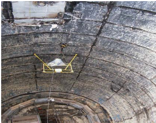
In-situ gamma spectrometry on steel containment
