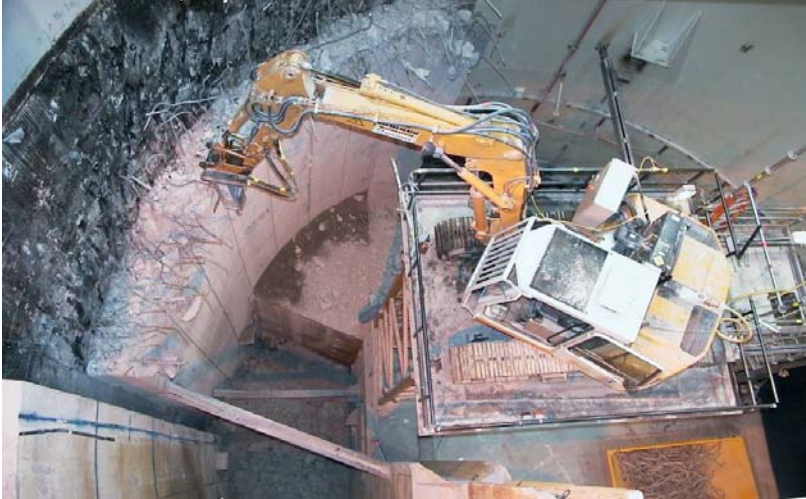
Removal by pneumatic rock excavator
