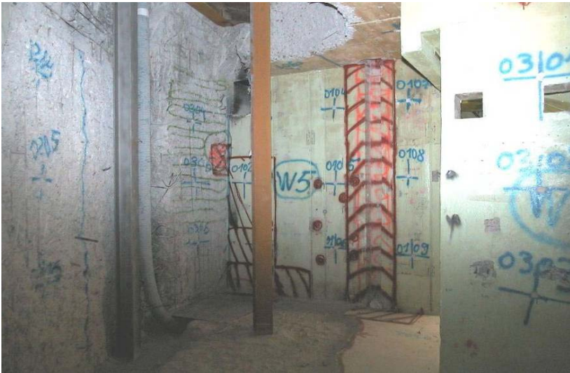
Marking of contaminated areas
