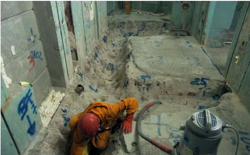
Removal by manual pneumatic hammer
