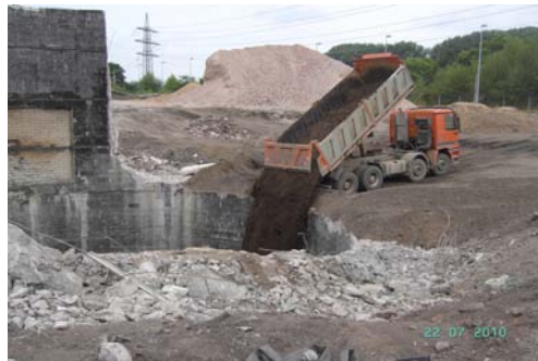
Filling reactor building pit below -4 m
