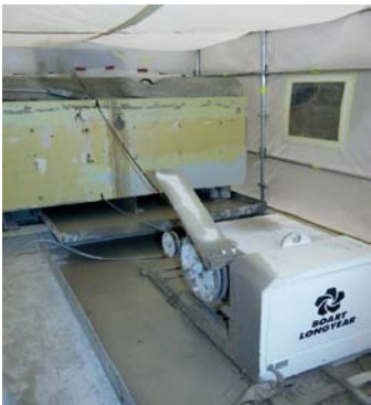
Removal by diamond wire saw
